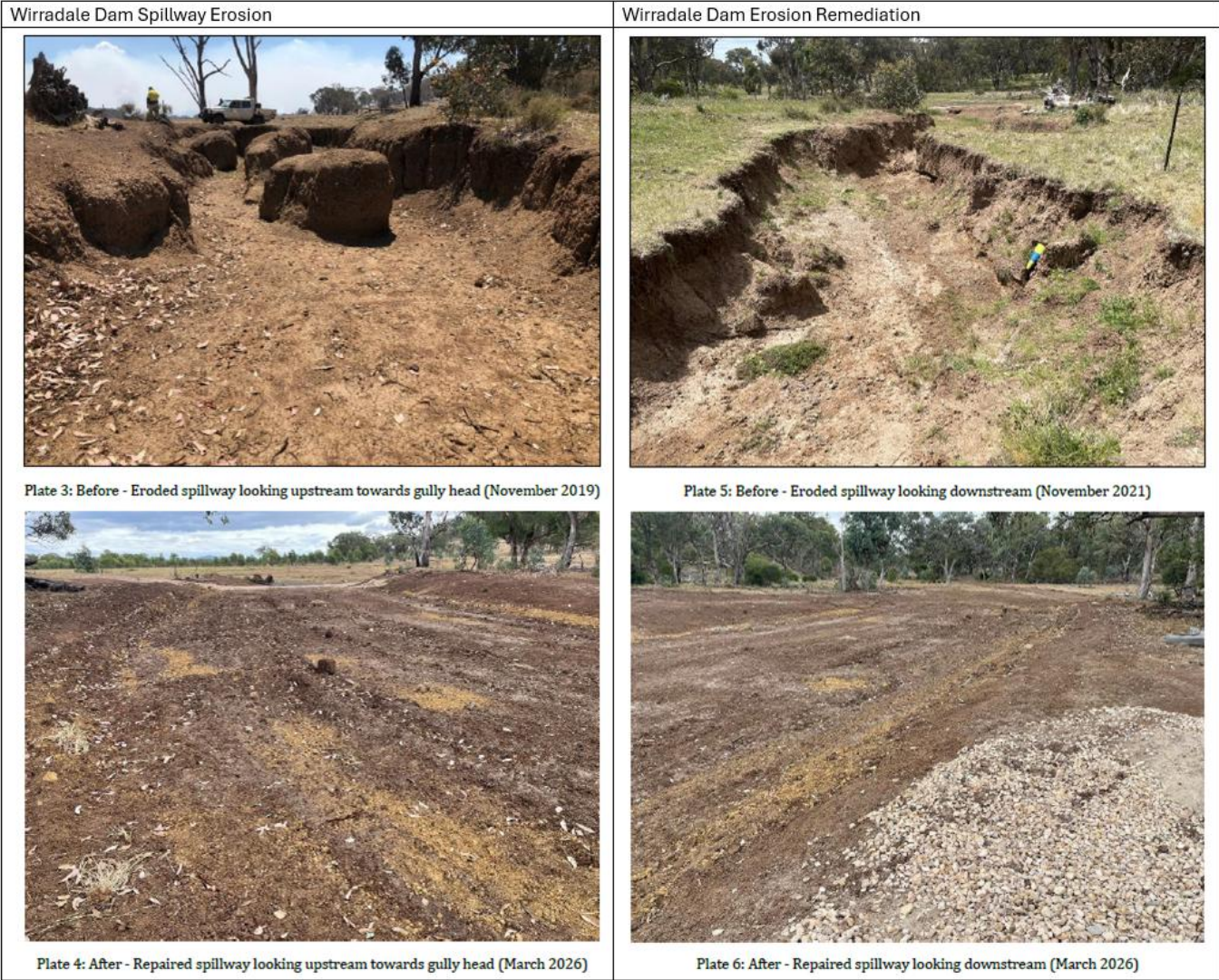
FIGURE 3-14 WIRRADALE DAME SPILLWAY EROSION REMEDIATION
