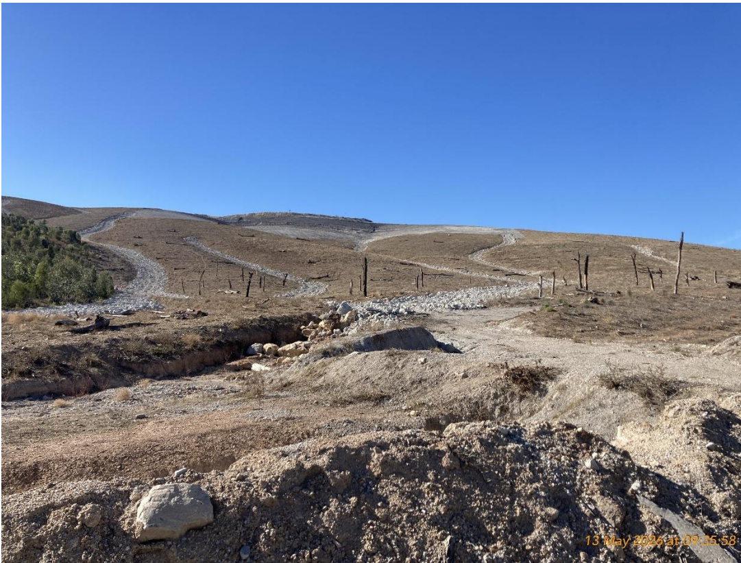
FIGURE 3-5 STAGS PLACED WITHIN RECENT REHABILITATION
